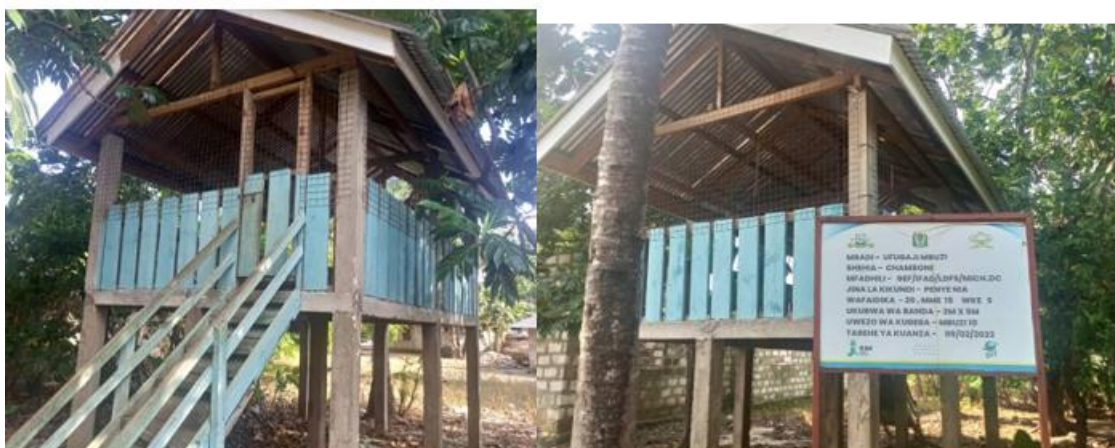
Plate 8: Upgraded Goat Sheds in Micheweni District that offers better ventilation, drainage, and protection from harsh weather conditions, ensuring a healthier environment for the animals
