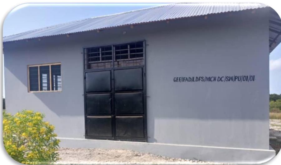
Plate 10: Sea weed processing facility at Shanake Micheweni District
