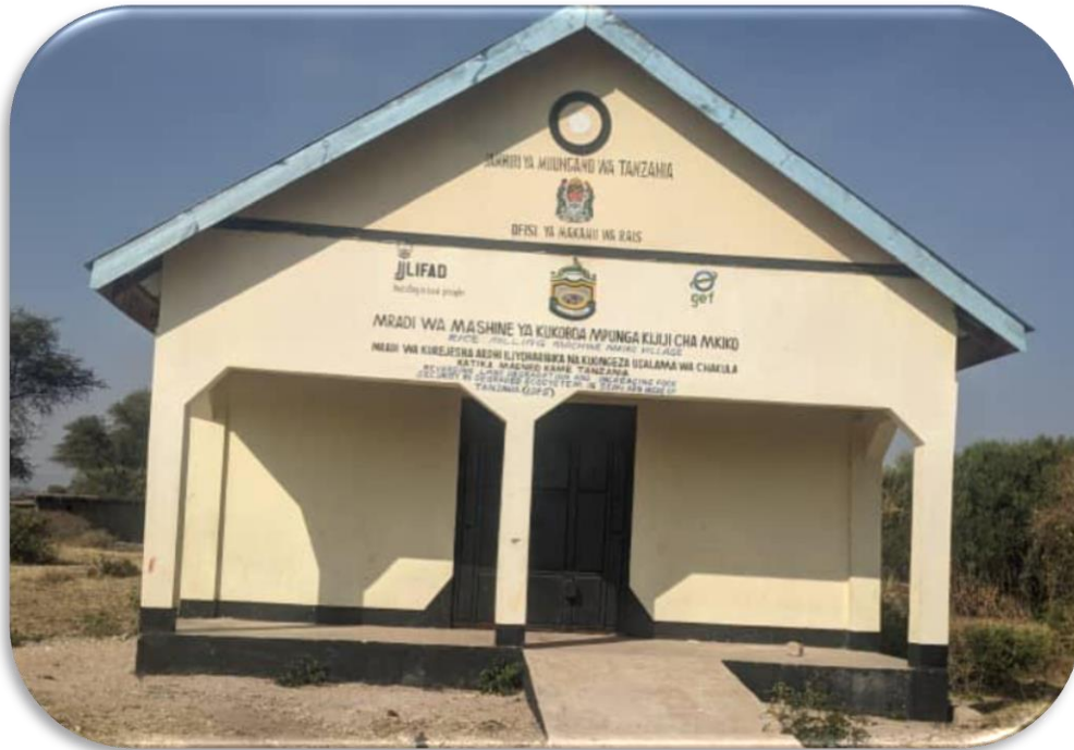
Plate 9: Rice processing facility at Mkiko village in Mkalama District
